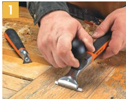
▲ For quick removal, use carbide scrapers to remove as much of the finish as possible ( see Sources, page 2 ).
