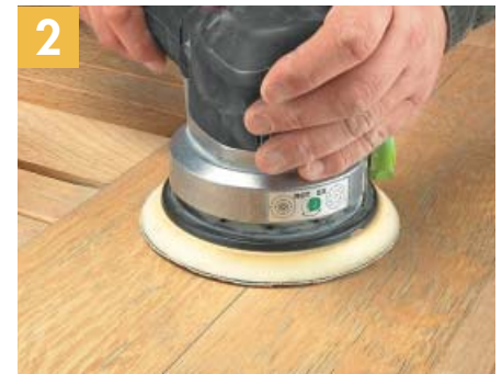
▲ After scraping, remove the rest of the finish from the wood by using 60-grit sandpaper on a random-orbit sander.
